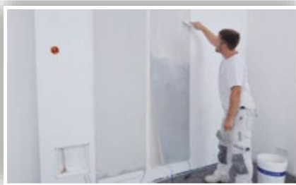
Glue the heating fabric.
